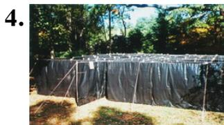
**Add rope supports as necessary** - When constructing long corridors, sometimes (depending on the design), the walls will become unstable and sag. If this is the case, stake a rope along the outside of the maze, and then run it over the top of the maze, and around the top of the maze panel struts which are sagging. This should stabilize the walls as necessary as you assemble the maze.
