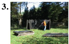
**Assemble the panels** - Using the diagram, assemble the panels. Start at one corner of the twine outline (see step #1) and then put panels together, connecting panels together by lining up the screw-eyes and then using cable ties to connect them together. See [this picture](#) for an example.
